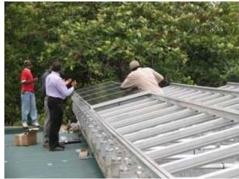
Figure 10: Installation of Solar Panels on the Roof of the SLNT
